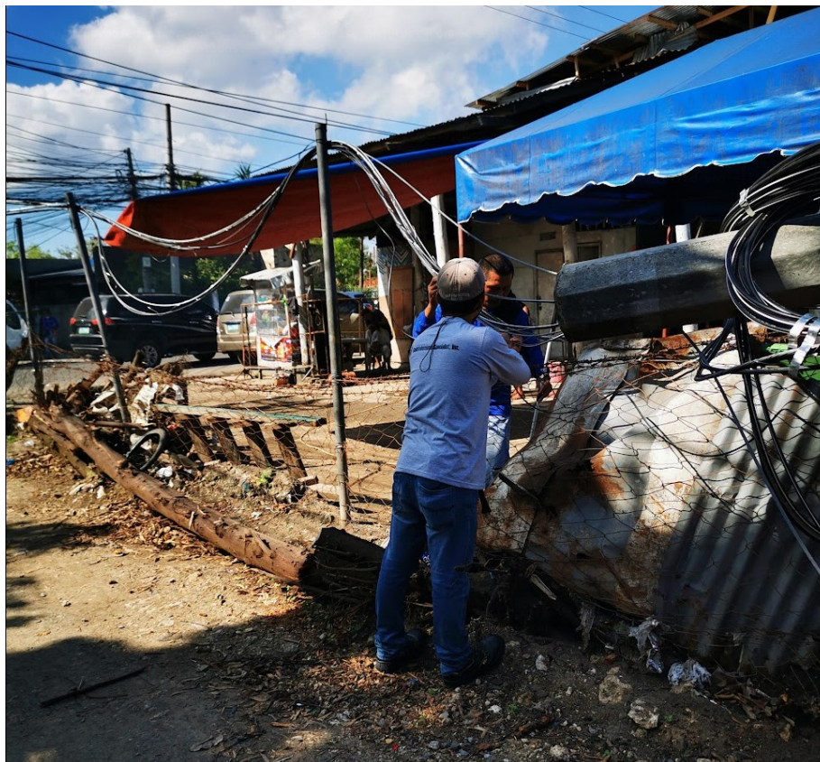
Figure 7. Steel columns are temporarily used for fibre attachment
