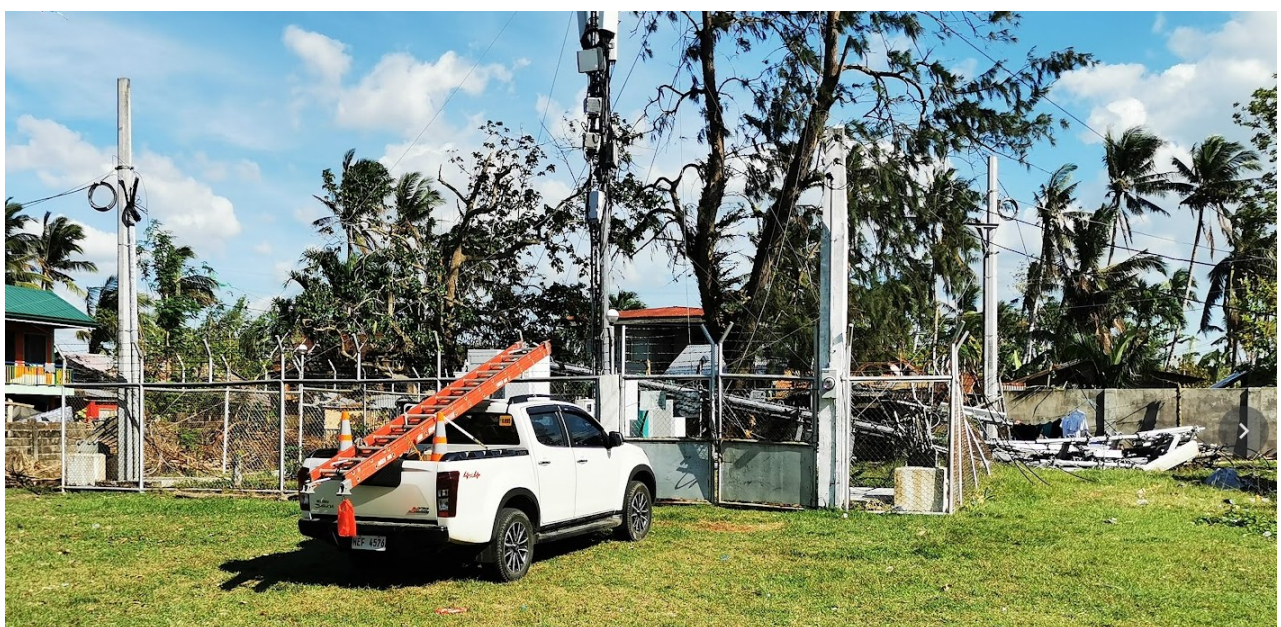
Figure 2. A toppled tower located somewhere near Toledo City
