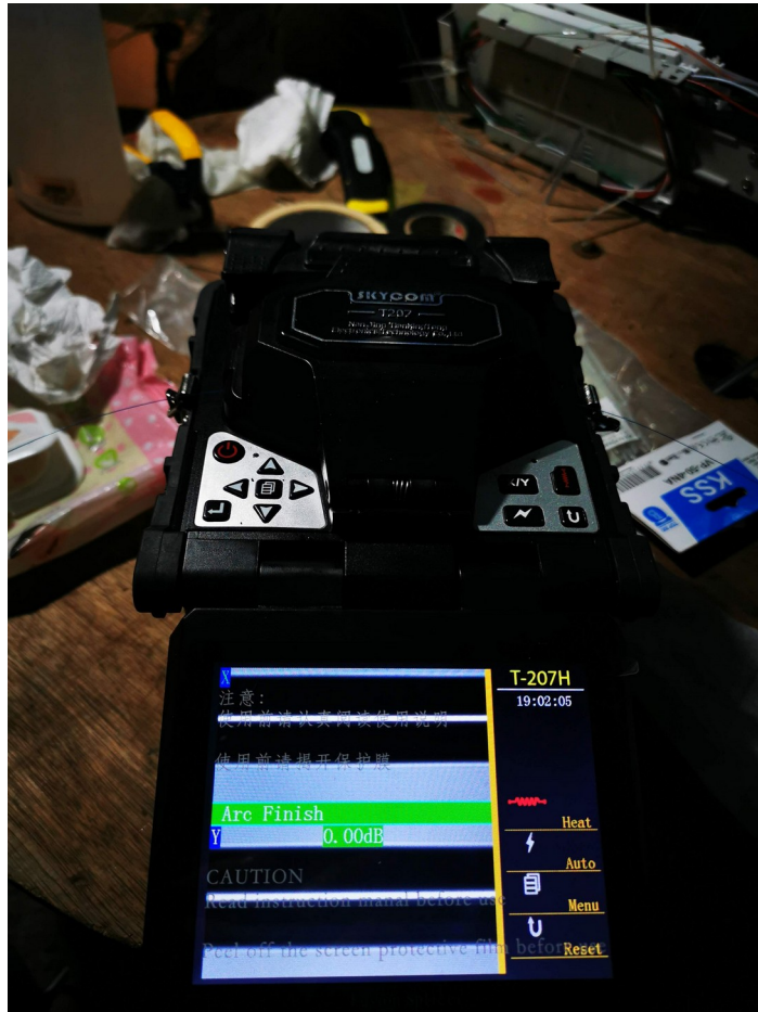
Figure 5. As seen on the OTDR display, I have just finished splicing the fibre.
