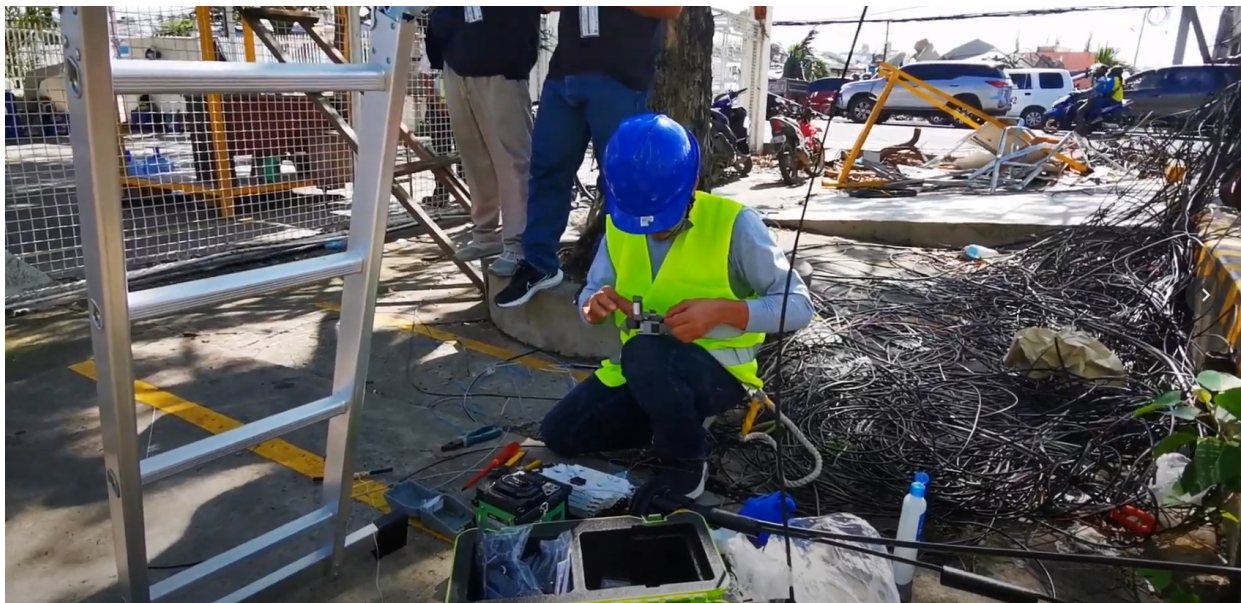
Figure 4. Preparation of fibre for splicing.
